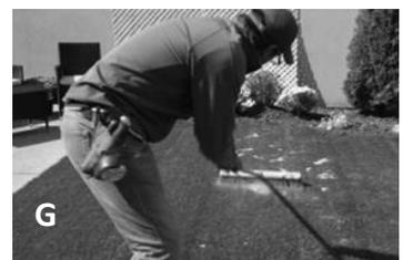
3. Use turf binder or outdoor adhesive to bind the artificial grass to the concrete slab, ensuring that you follow the manufacturer's directions.
